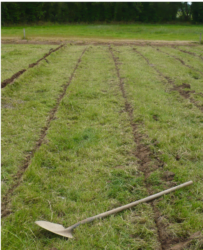
Figure 5- A mole drain with 4-ft spacing. Note that the 4-ft spacing may result in the desired spacing of 8 ft or wider assuming some of the mole channels will fail (Photo credit: Patrick Tuohy)
